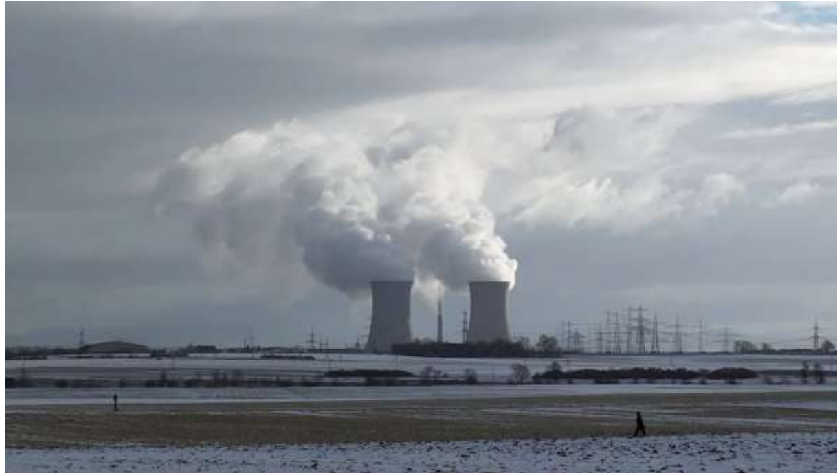
Cooling water Cooling towers
